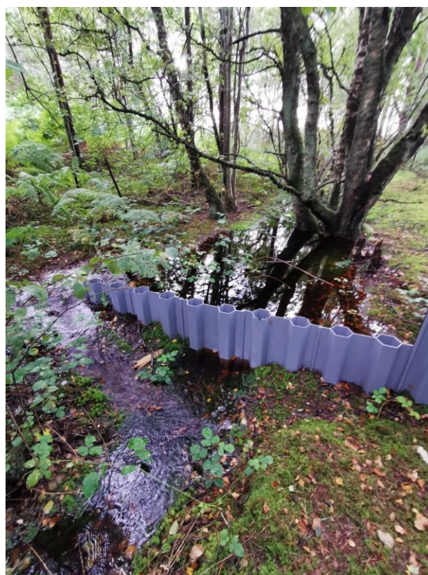
Figure 5.8 Example of targeted blocking of drains with plastic dams in densely wooded areas
