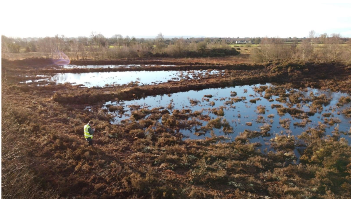
Figure 5.6 Example of cell bunding completed at Clara Bog SAC
