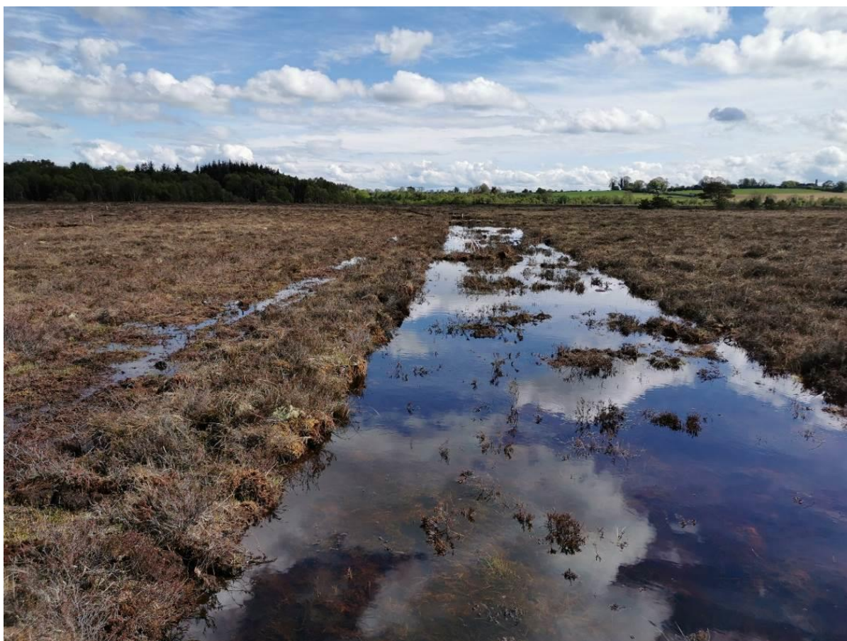
Figure 2.3 Example of a contour bund constructed at Knockacoller Bog SAC, Co Laois
