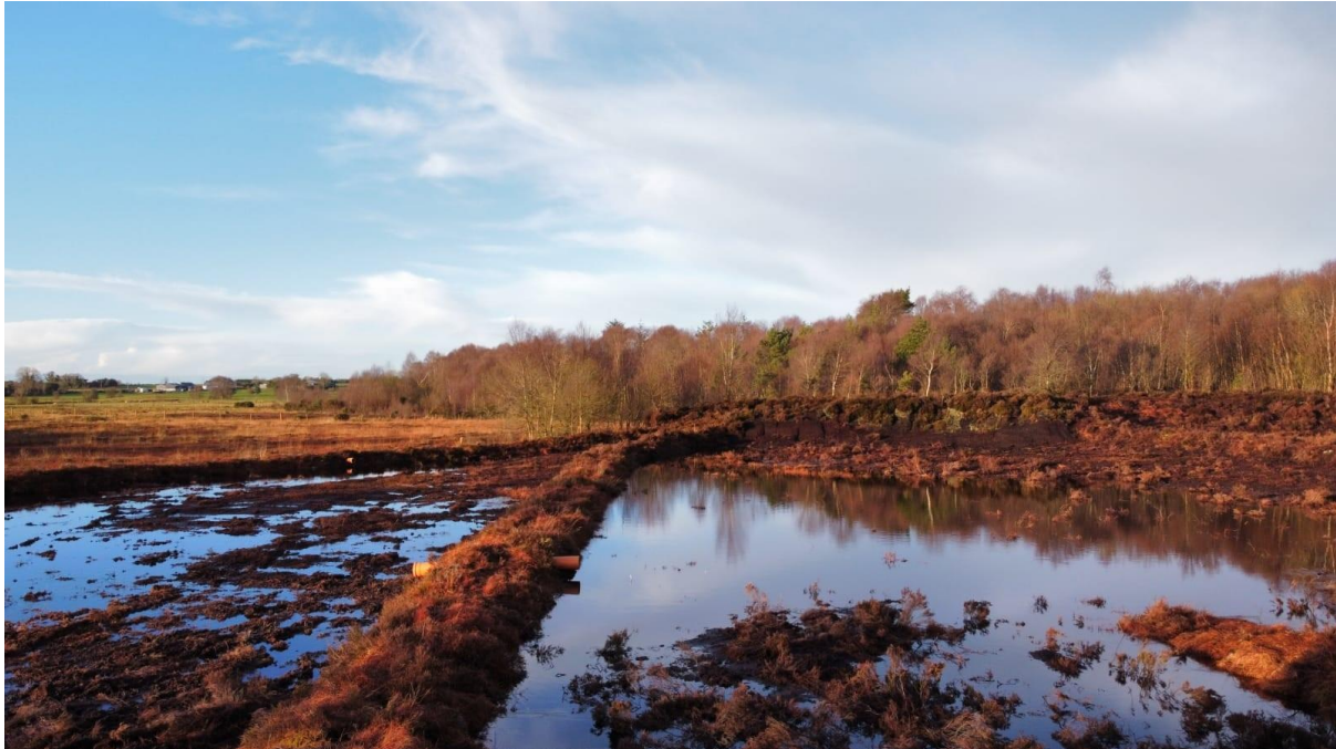
Figure 2.4 Example of existing cell bund constructed at Cloncrow Bog NHA
